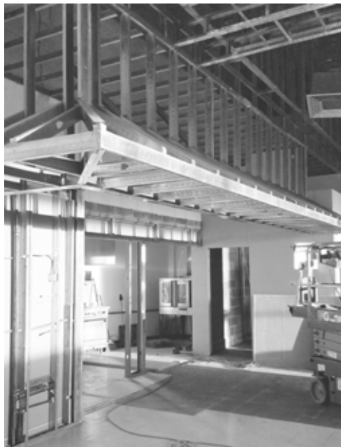
The new awning which will house recessed lighting is taking shape.
